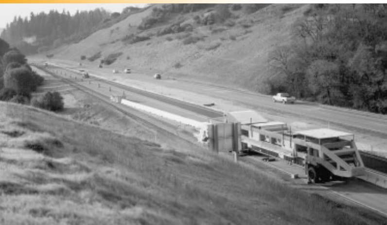
The Pavement Research Center's Heavy Vehicle Simulator testing pavement on U.S. 101 near Ukiah, CA
